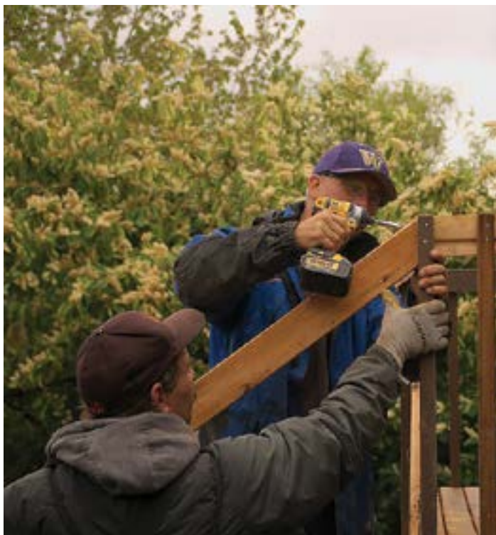
RTS volunteers collaborate to fix a handrail.
